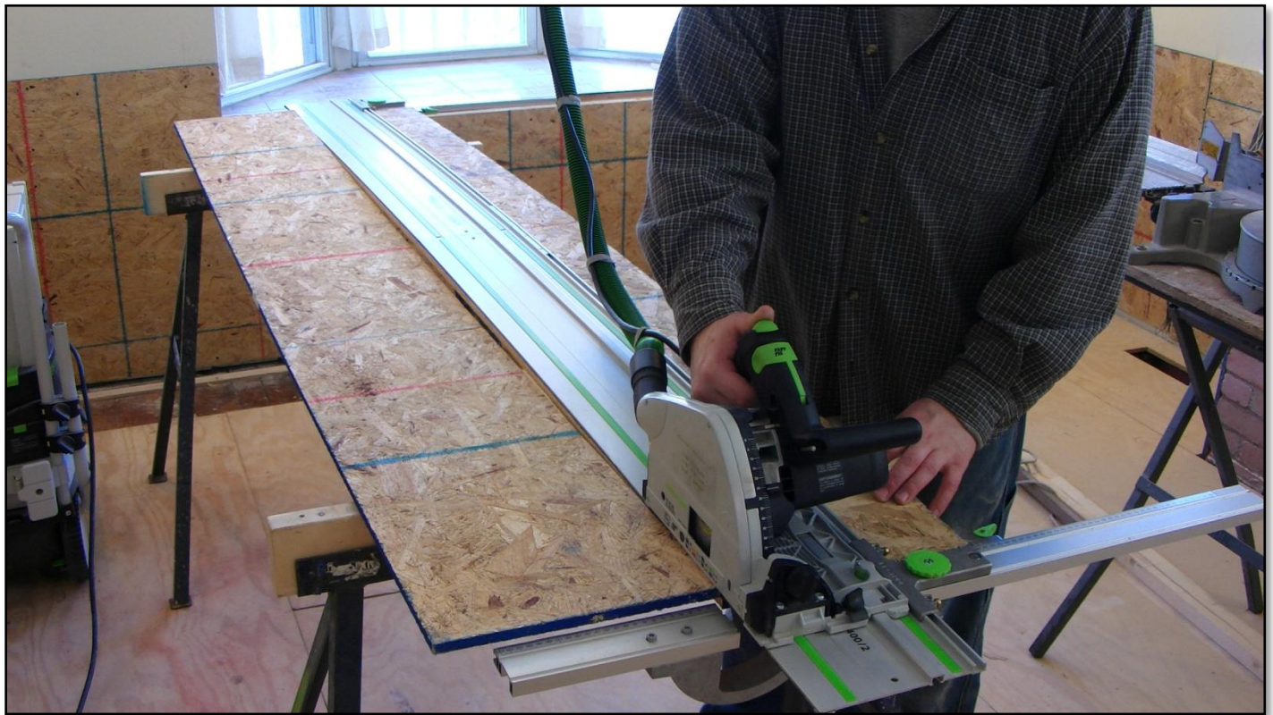
Here I'm making a rips on a sheet of OSB for a backing to wainscoting.
